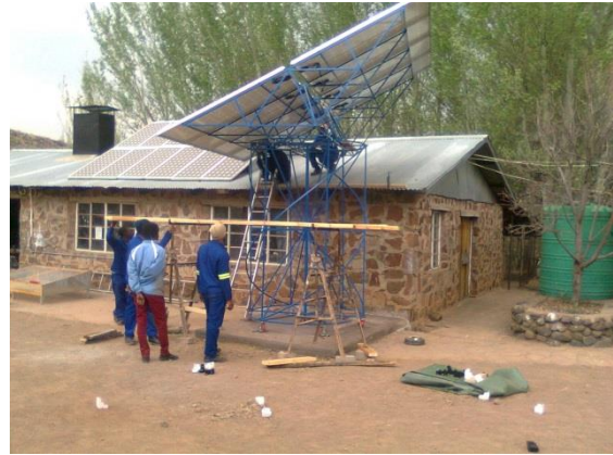
Fig. 29: 2.5KW solar array for water pumping being assembled on BBCDC campus, Sept.
