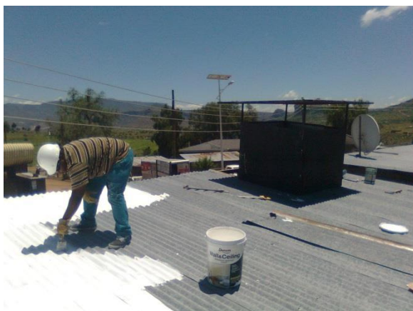
Fig. 3: Cool roof installed in Mt. Moorosi: white paint and solar chimney, Jan.
