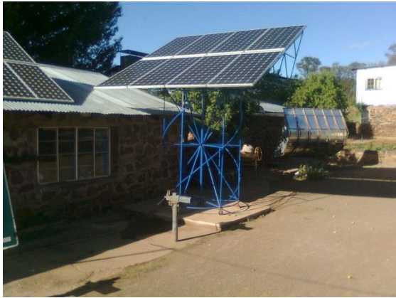
Fig. 44: 2.5KW array rotating to capture sun all day and pump water for 12 hours, Nov.
