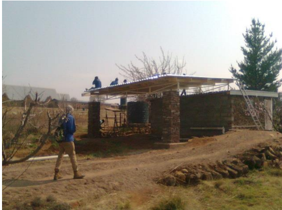
Fig. 27: Columns and roof for vehicle park on BBCDC campus, Aug.
