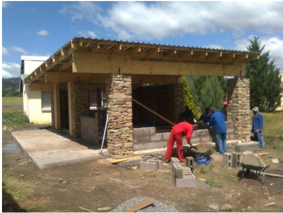
Fig. 14: Infill walls being built new workshop Mohales Hoek, March.
