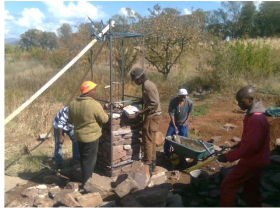
Fig. 17: Construction of two columns for vehicle parking garage at BBCDC, April.
