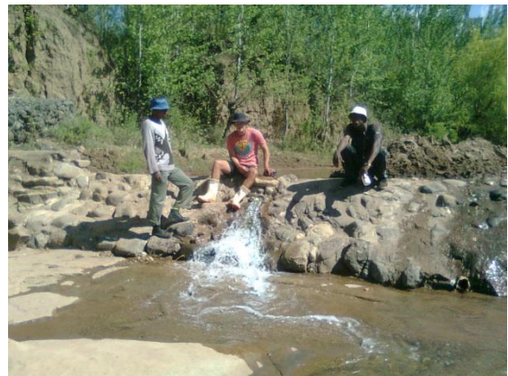
Fig. 43: releasing stored water behind ground water dam for irrigation, Nov.
