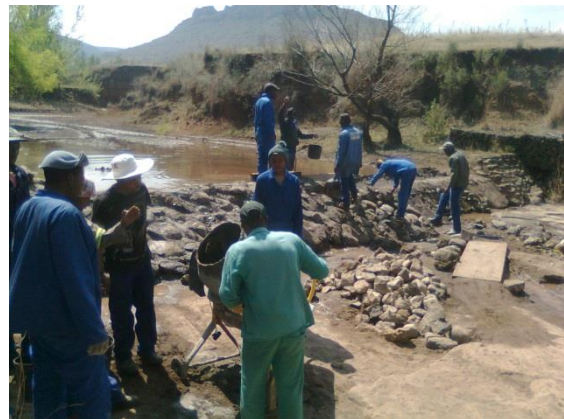
Fig. 31: Construction activities to raise ground water dam wall with stones and mortar, Sept.
