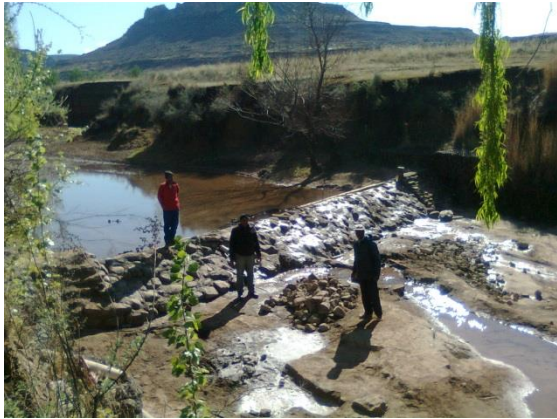
Fig. 32: Ground water reservoir filled with coarse sand after heavy rain event, Sept.
