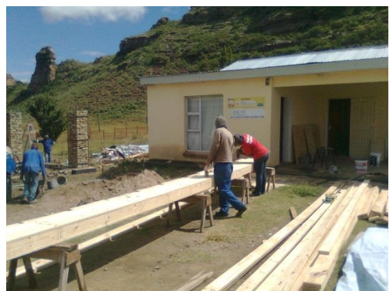
Fig. 12: Box beams and rafters being built for new workshop, March.
